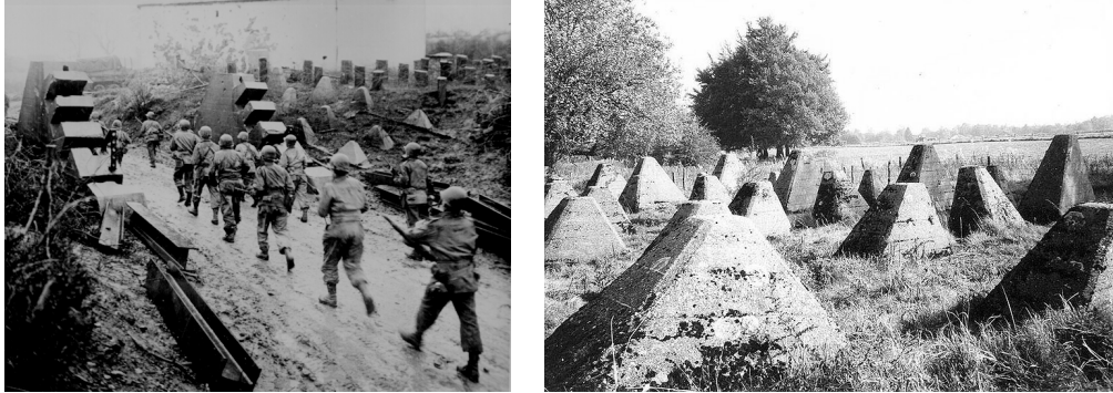
Figure 4.9: The Siegfried Line was built during the 1930s. The Germans themselves called this the Westwall, but the Allies renamed it after the First World War line. The Siegfried Line was a defense system stretching more than 390 miles with more than 18,000 bunkers, tunnels and tank traps. It went from Kleve on the border with the Netherlands as far as the town of Weil am Rhein on the border to Switzerland. Adolf Hitler planned the line from 1936 and had it built between 1938 and 1940. LEFT: Americans crossing the Siegfried Line into Germany. RIGHT: “Dragon’s teeth” tank traps on the Siegfried Line.
