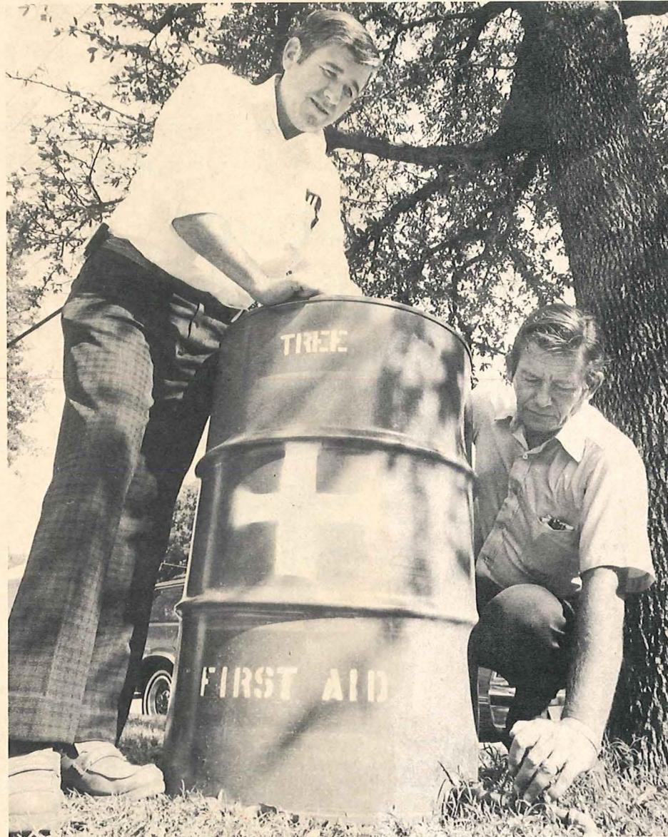
Pluenneke designed a portable trickle irrigation system to help trees during the hot, dry North Texas summer. It aids trees outside the normal irrigation system.
