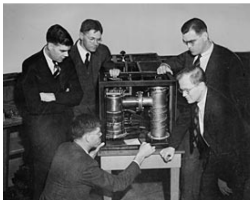
Figure 48. Researchers examine the first klystron at Stanford University in 1939. Standing L to R Sigurd Varian, David Webster, William Hansen. In front, Russell Varian and John Woodyard, Washington alumnus. (Stanford News Service photo)
