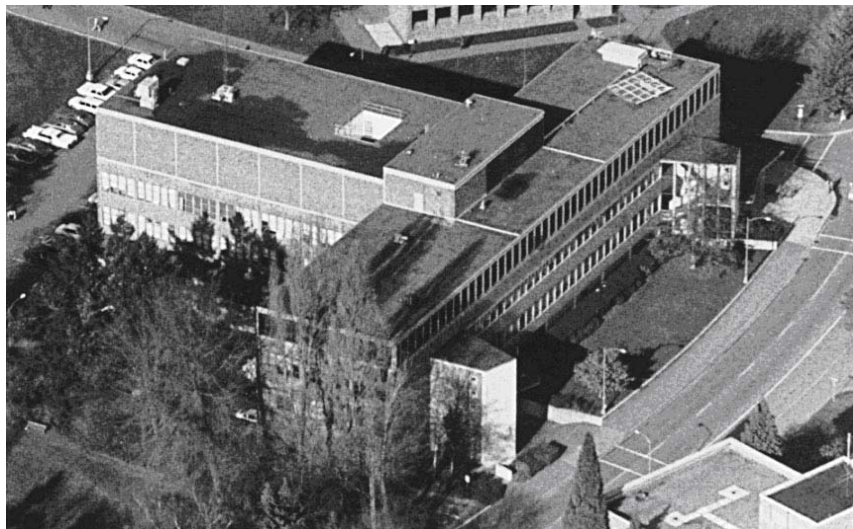
Figure 92. The Electrical Engineering building in the 1960s, after construction of the fourth floor. The indoor antenna range occupied the windowless space in the base of the T. (EE Department photo)
